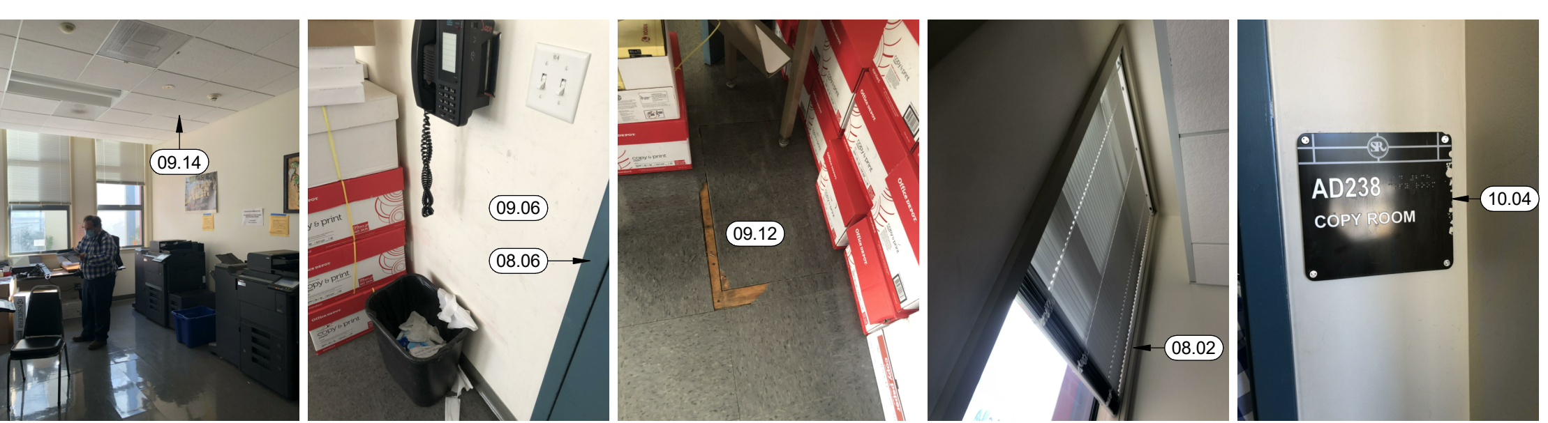
19 COPY ROOM REPAIR PHOTOS 1/8" = 1'-0"
